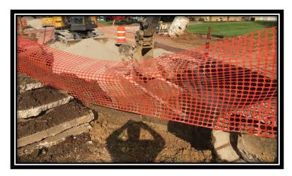
After observing employees of Legacy Corporation of IL performing work in the City of Moline, <u>IL</u>, III FFC employee Andrew Waeyaert filed an OSHA complaint alleging that employees working in a trench box were exposed to crushing injuries because the trench box was not secured from movement in the
